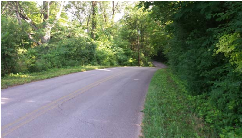
View at Proposed Entrance Road “K” at Sam Lee Road (Looking “East”)
