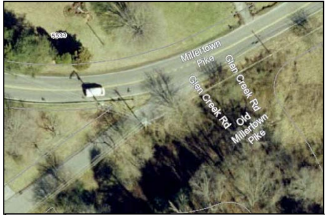
View of Old Millertown Pike at Millertown Pike prior to re-alignment (KGIS, 2003 Aerial Map)
